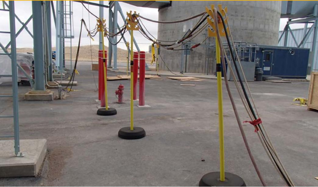
RubberForm's Portable Electric Cable Support Tower (PECST) is a portable cable support engineered by safety and construction workers after the realization that traditional wooden cable trees were unsafe and inefficient. Our PECST's are made with our durable rubber base and fibre-reinforced plastic poles and antlers which make them completely non-conductive.
