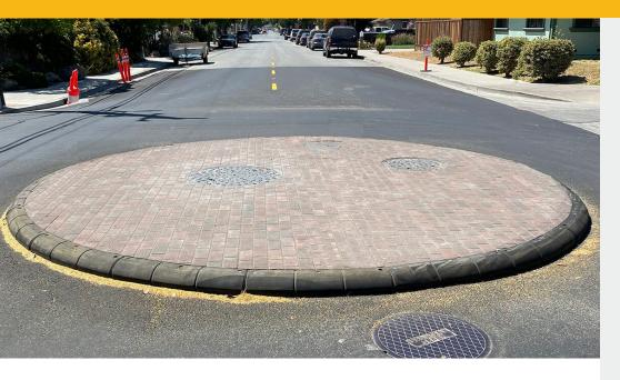
The RubberForm Engineered Rubber Curb is a temporary or permanent curbing solution manufactured from heavyduty recycled rubber. They offer a superior performance that easily outlasts concrete with hard-wearing durability and low maintenance.
