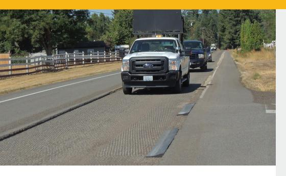
RubberForm's Wedge Ramp is an efficient and sustainable alternative to cutting into curbs or as a replacement for temporarily laying down gravel or asphalt for transition over sunken pavement or other uneven surfaces during construction projects.
